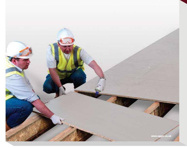
The Rapid Deck Floor Laying System involves bonding EGGER Protect board to the joists and into the tongue and groove of the board using EGGER D4 Adhesive. Designed primarily to reduce installation times and also minimise squeaking floors, whilst complying with current HSE regulations for floor decking.
